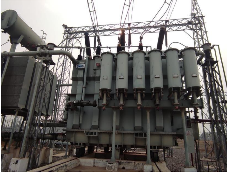
Figure 7: Power transformer
