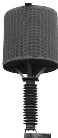
Figure 8: Wave Trap
